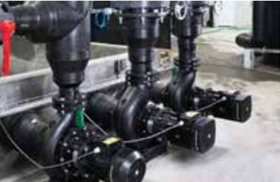
Multi-purpose end-suction pump is an ideal solution in oxygen cones and can also be applied in CO 2 degassing.
