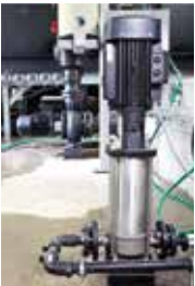
Multi stage centrifugal pump A perfect wash down pump for drum filter cleansing. Flow propeller pump Designed for CO 2 degassing.
